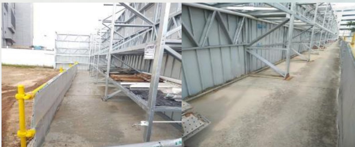
Clean & Unobstructed Site Access/Entry
