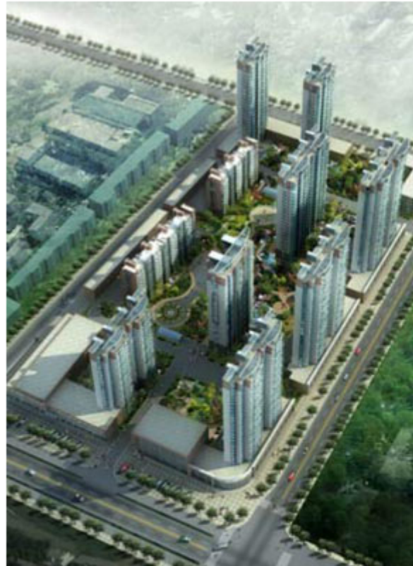
Tiong Seng's mixed residential / commercial development project in Cangzhou, China: Cangzhou Sunny International Project
