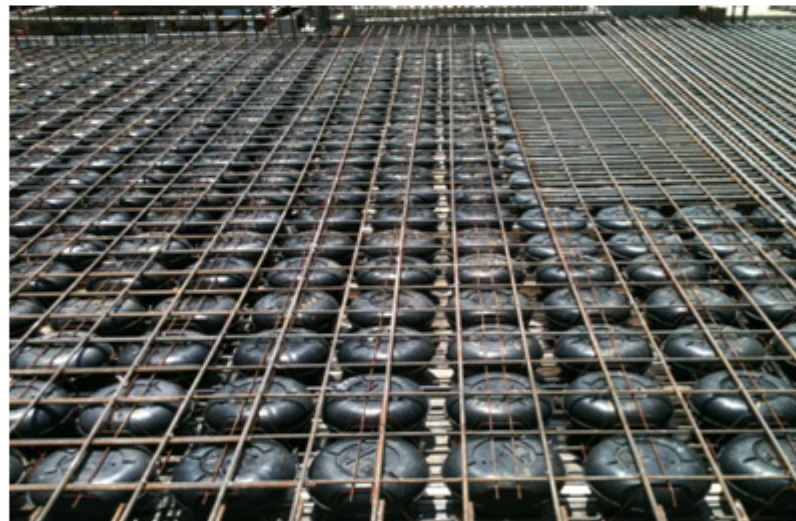
Cobiax balls encased in steel mesh: With the balls in place, less concrete is needed in the production of slabs.
