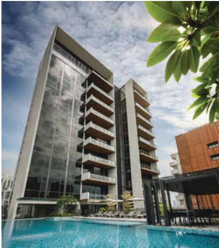
Sloane Residences Client: TSky Balmoral Pte Ltd Approx Contract Value: S$28.9 million
