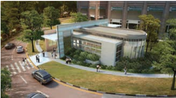
Contract T220 – Great World Station Client: Land Transport Authority Approx Contract Value: S$324.0 mil
